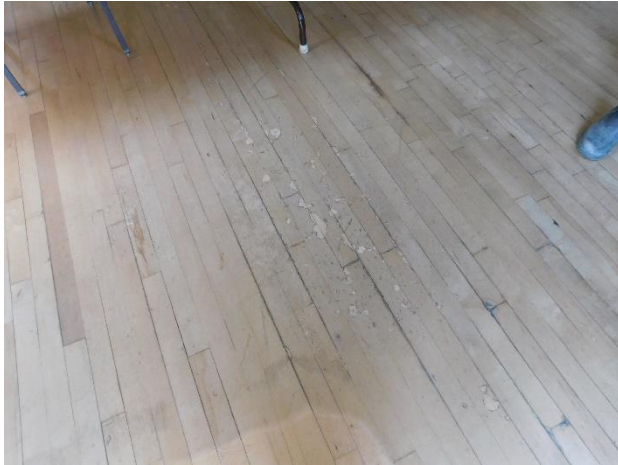
Figure 79. Peeling floor finish in the main hall.
