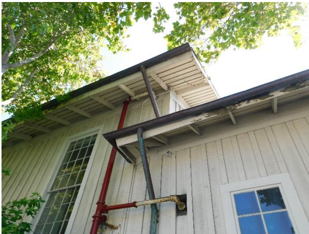
Figure 48. Copper gutters and rain leaders.
