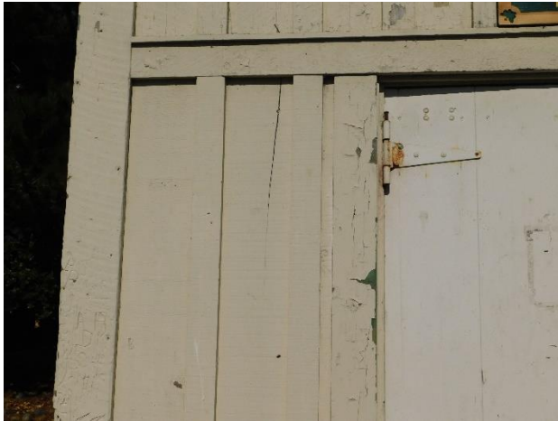
Figure 27. Example of splitting board and batten cladding.
