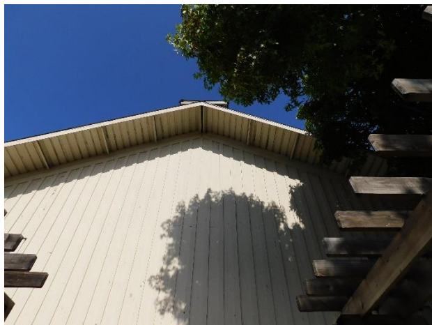
Figure 23. Typical board and batten siding.
