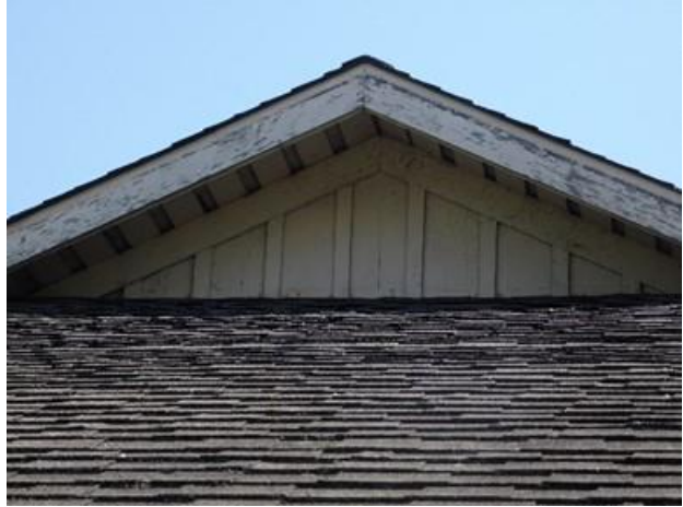
Figure 47. Example of painted barge boards at gable ends.
