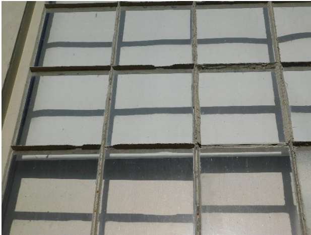
Figure 37. Example of damaged or missing muntins. Note also the cracked and missing glazing putty.
