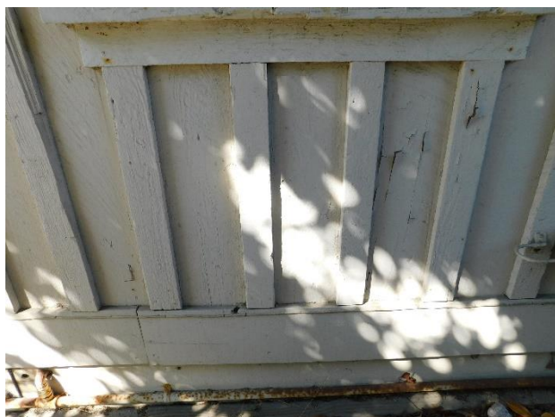
Figure 25. No metal flashing at water table along south facade of ancillary spaces (line near top of water table trim is a small wire). Also note the loose and peeling paint.
