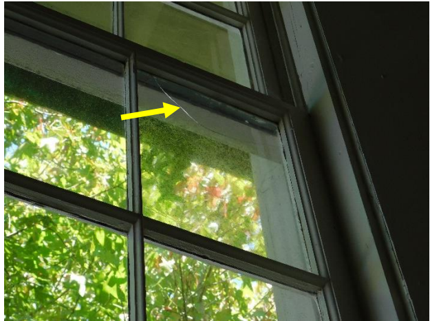
Figure 38. Example of cracked window lite (arrow).
