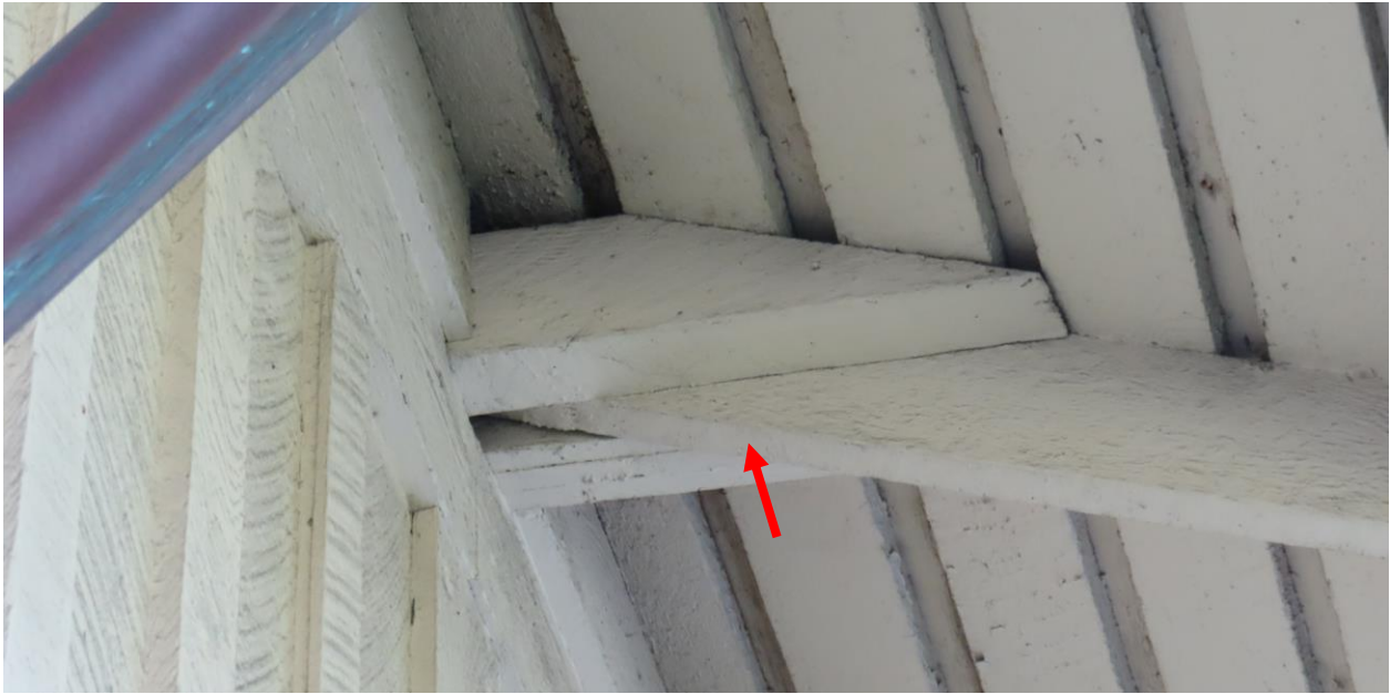
Figure 86. Heel connection of truss just outside the exterior wall of the main hall (arrow).
