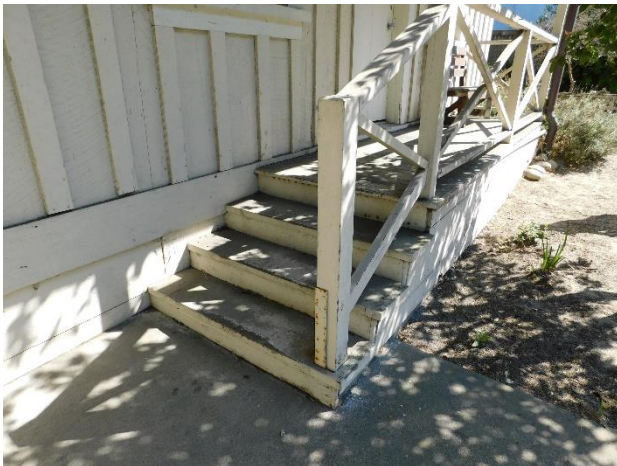
Figure 18. Porch with loose guard rail post.
