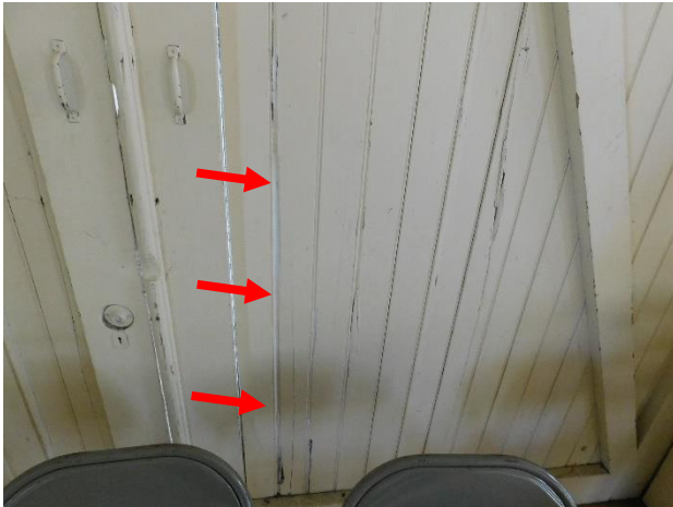
Figure 45. Previous sealant repairs at the large-double leaf doors on the east facade. Also note the daylight visible between the stile and the bead boards.
