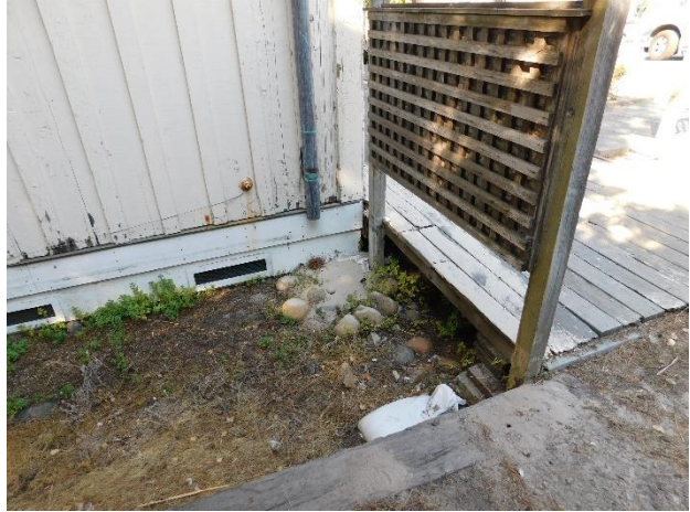
Figure 59. Example of typical rain leader discharging adjacent to the building and its foundation.
