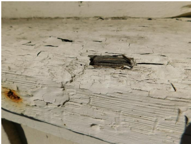
Figure 35. Example of isolated areas of wood deterioration at wood sills.
