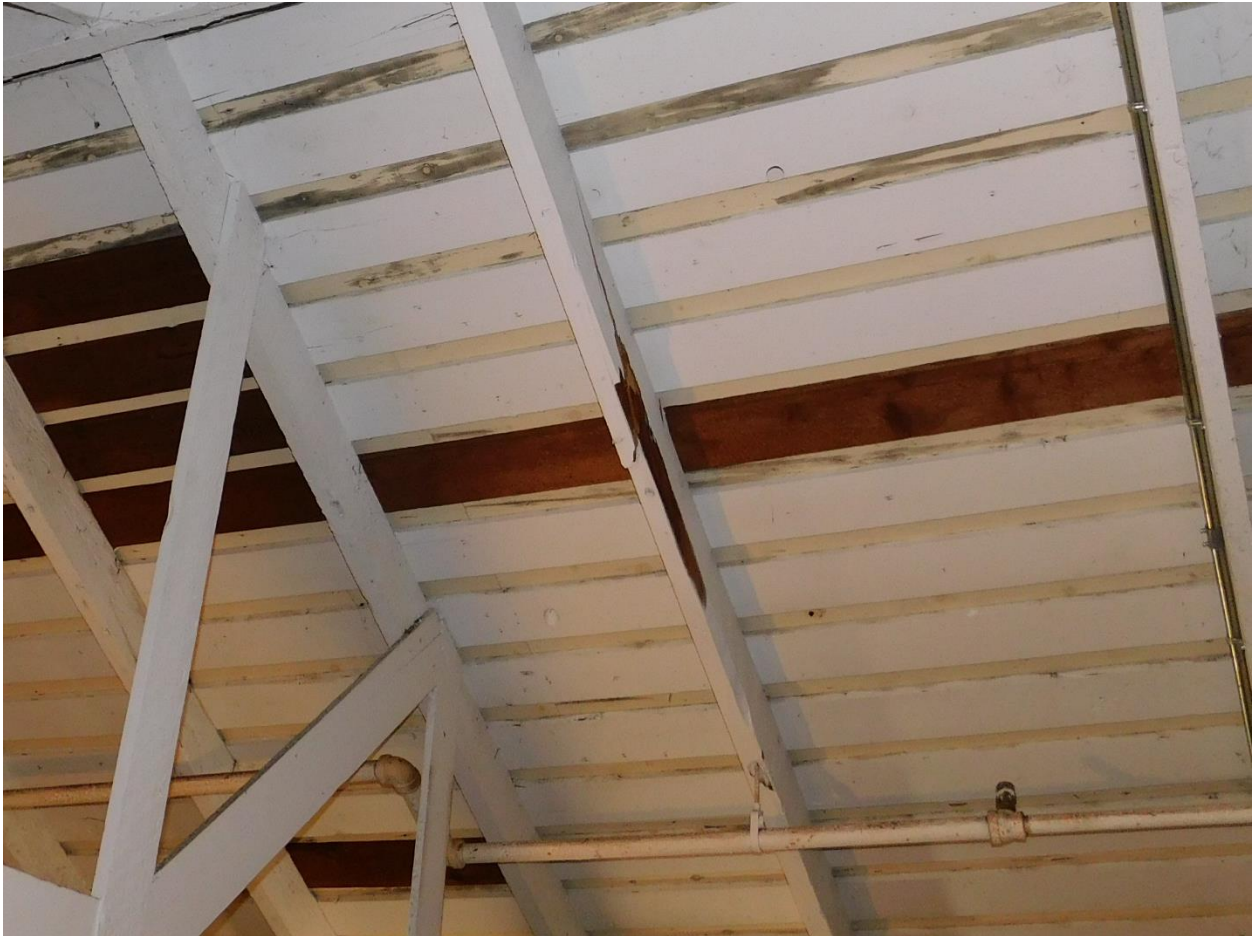
Figure 91. Fractured roof rafter in the main mezzanine.
