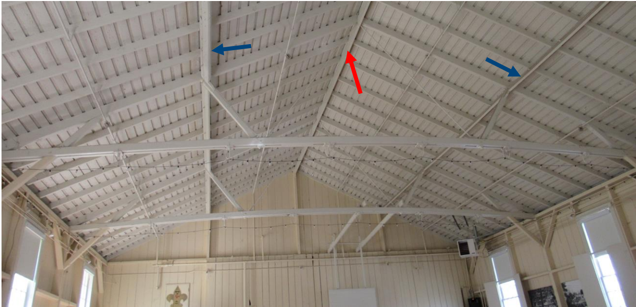
Figure 84. Roof system in the main hall. A ridge beam (red arrow) and strong backs (blue arrows) support roof rafters and span between trusses.
