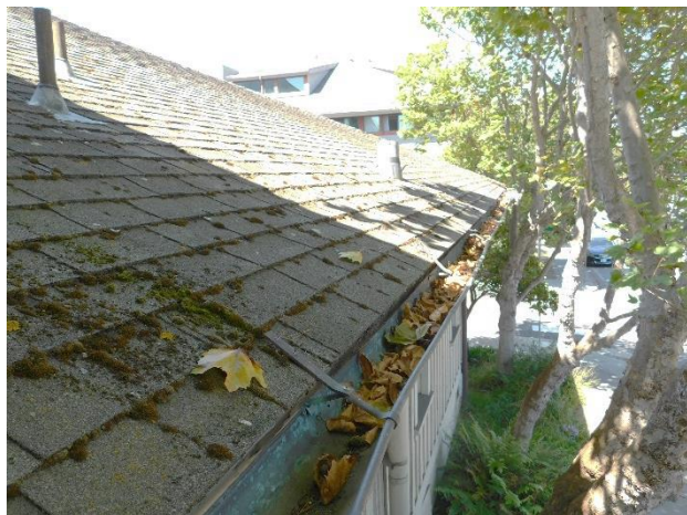
Figure 54. Debris collecting in gutters, exposed and loose fasteners, and bent gutter spacers.
