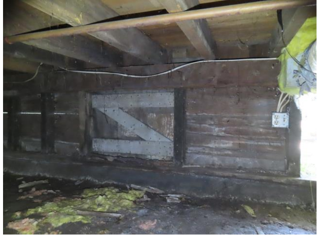
Figure 90. Exterior cripple wall framing
