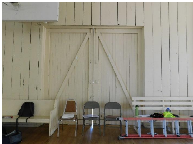
Figure 39. Example of a framed-and-braced exterior door at the large double-leaf doors on the east facade.
