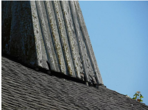
Figure 63. Detail view of deterioration at the base of the belfry.
