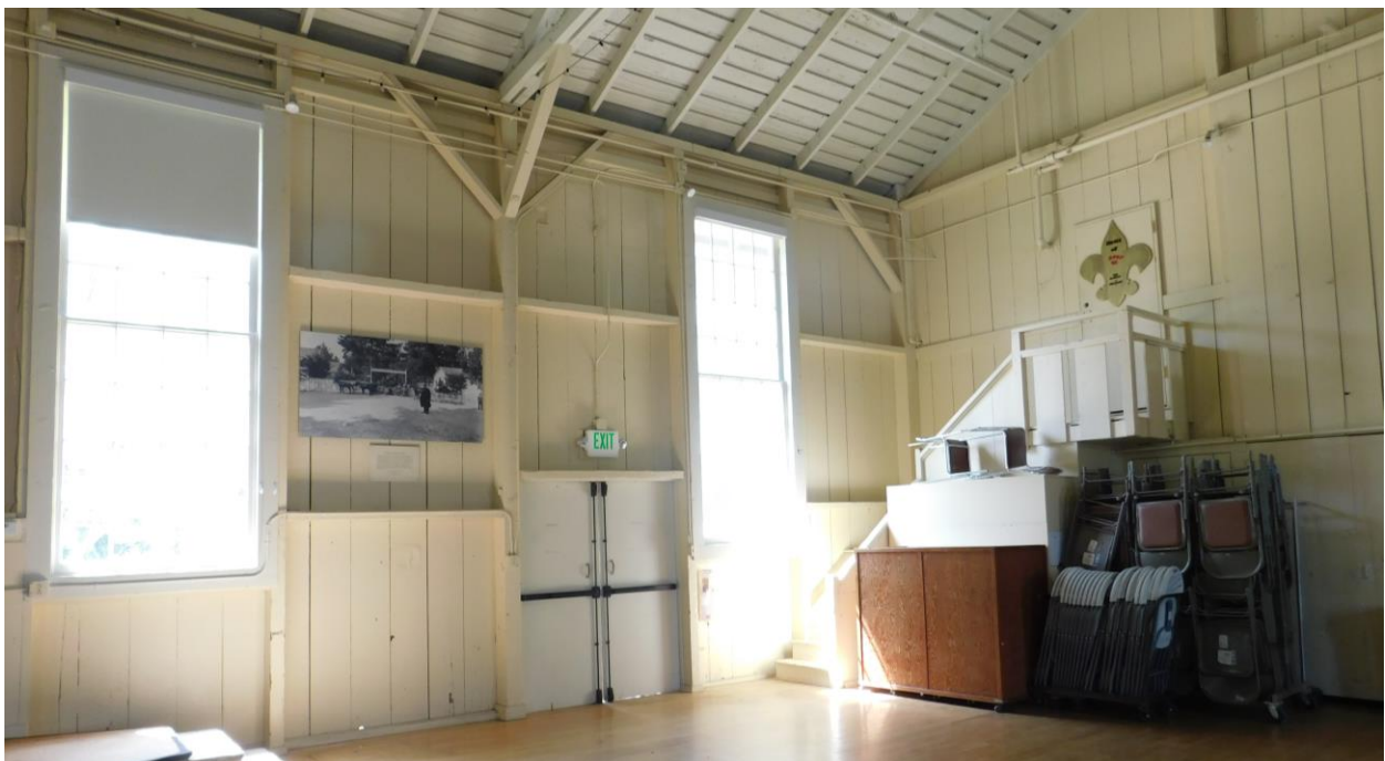
Figure 87. Typical wall framing in main hall.
