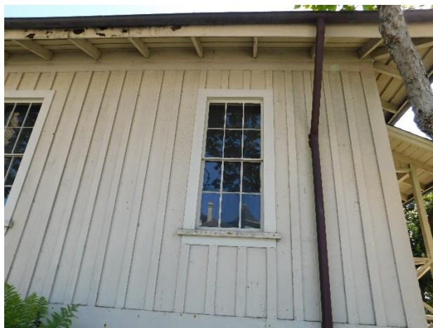
Figure 30. Original 6/6 double-hung wood window at one of the west multipurpose corner rooms.
