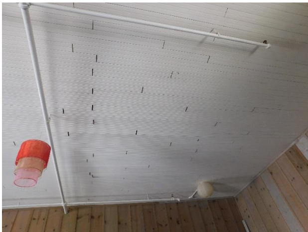
Figure 81. Large gaps between ceiling boards in the northwest multipurpose room.
