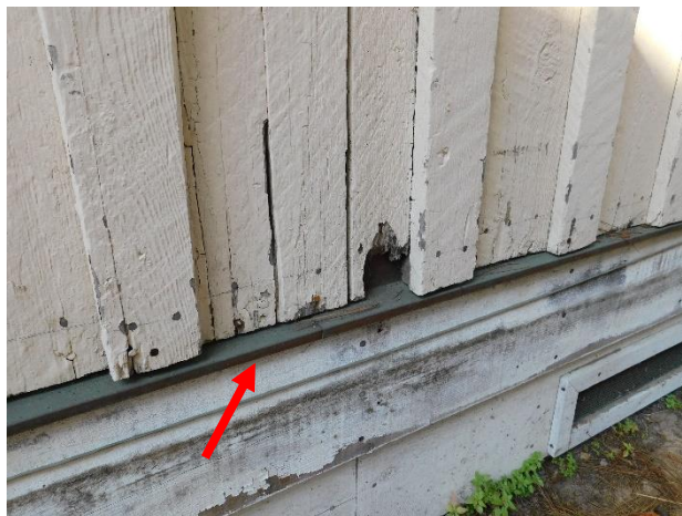
Figure 24. Metal flashing (arrow) at water table on south facade of main hall.
