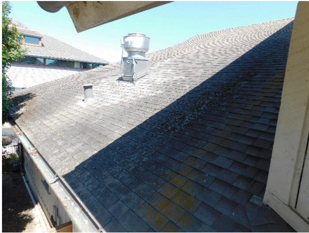
Figure 50. Condition of the roof over ancillary spaces.
