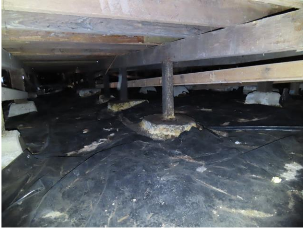
Figure 89. Typical joists, beams, and posts supported on shallow concrete piers.
