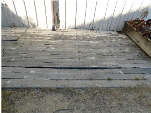
Figure 17. Sagging deck boards at the south deck.
