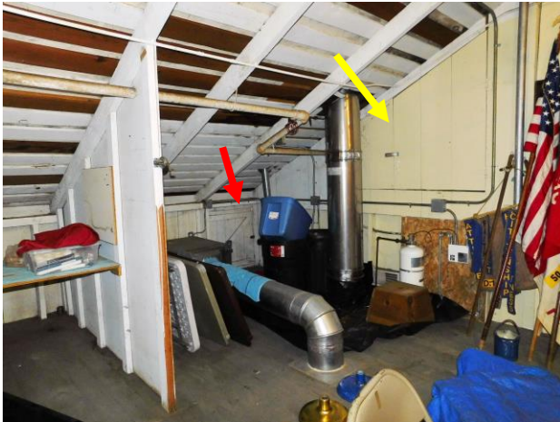
Figure 70. View of the main mezzanine looking south. Note the exposed kitchen ventilation ducts. Note the small hatch to the eave (red arrow) and the access door to the attic space above the multipurpose rooms (yellow arrow).
