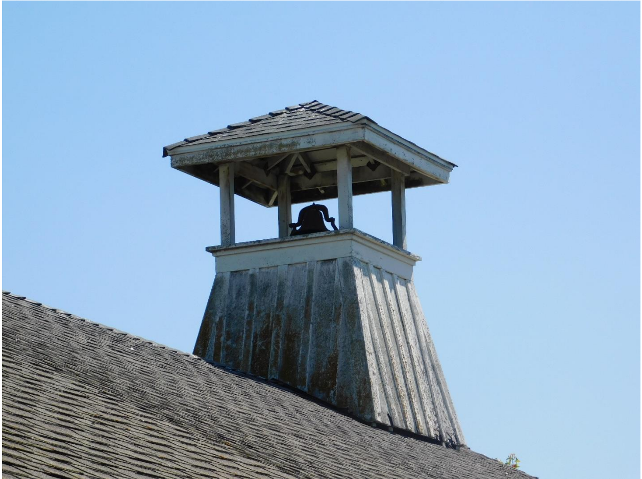
Figure 61. View of the belfry from the southwest. Note the significant biological growth on the west facade.
