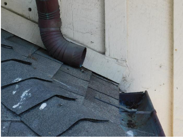
Figure 58. Missing kickout flashing at south wall of main hall. Also note the exposed roofing nails at the hip shingles.
