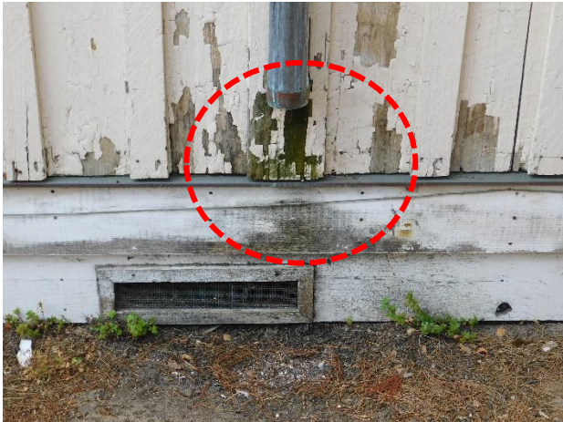
Figure 60. Example of a rain leader discharging high above grade. Note the greater amount of biological growth, wood deterioration, and paint loss around this area (dashed red line).
