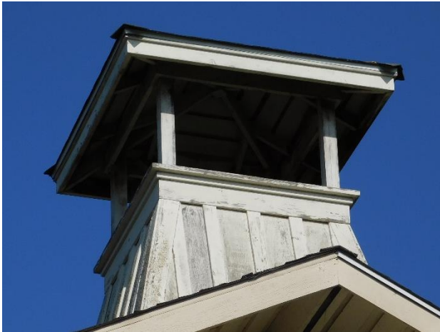
Figure 62. Detail view of missing, weathered, and peeling paint.
