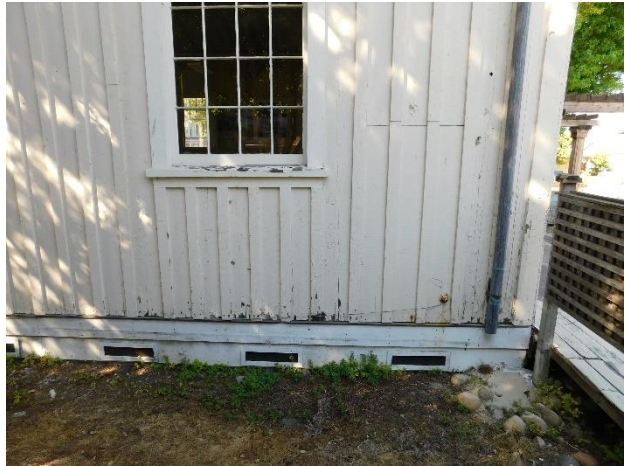
Figure 28. Example of deteriorating board and batten cladding at base of the wall.
