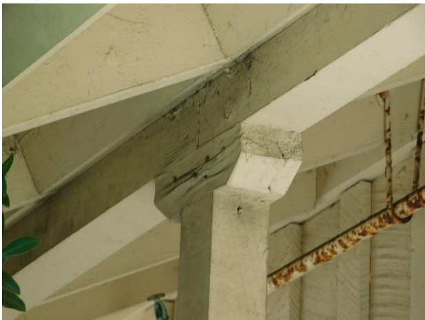
Figure 20. Crushing at corbel at west porch.
