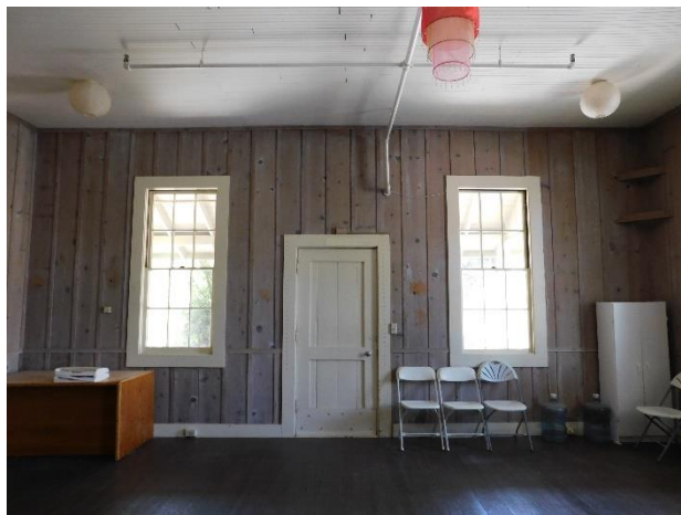
Figure 40. Example of a framed-and-ledged door at the west facade.
