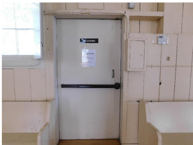
Figure 41. Example of a flush door with emergency exit hardware at the main hall.
