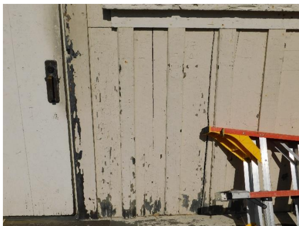
Figure 26. Example of weathered and peeling paint typical throughout the cladding. Also note the splitting boards.
