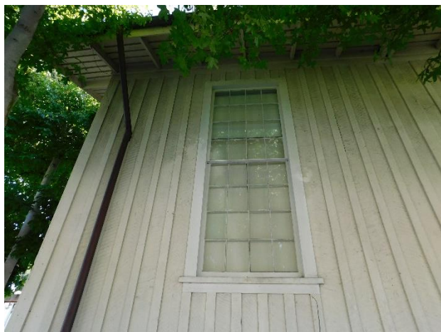
Figure 29. Original 8/8 double-hung wood window at the main hall.
