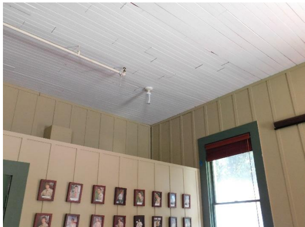
Figure 82. Smaller gaps between ceiling boards in the southwest multipurpose room.
