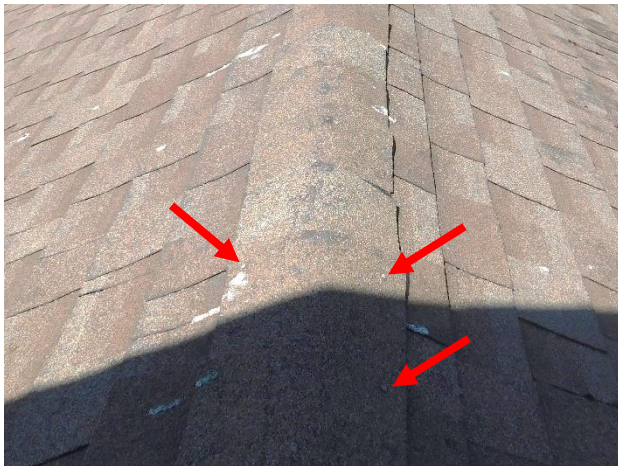
Figure 52. Exposed fasteners (arrows) and unfavorable direction of lap of ridge shingles at roof over ancillary spaces.
