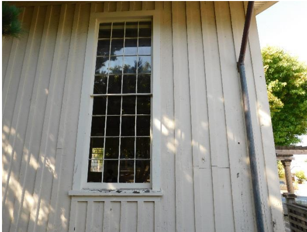
Figure 33. A south window of the main hall in serviceable condition with peeling paint at sills.
