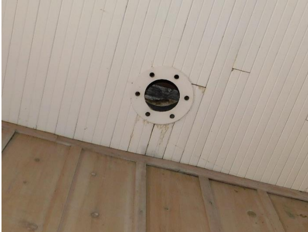
Figure 83. Water staining around abandoned vent in the northwest multipurpose room.
