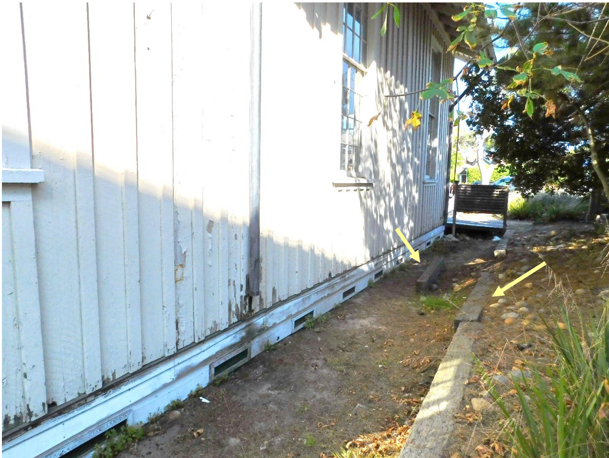
Figure 6. View of the short retaining wall along the south facade of the main hall. Note also the rotated and displaced retaining wall timbers (arrows).
