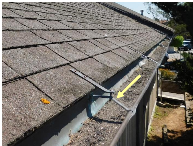
Figure 55. Exposed gutter strap fasteners through roofing and bent gutter spacers (arrow).
