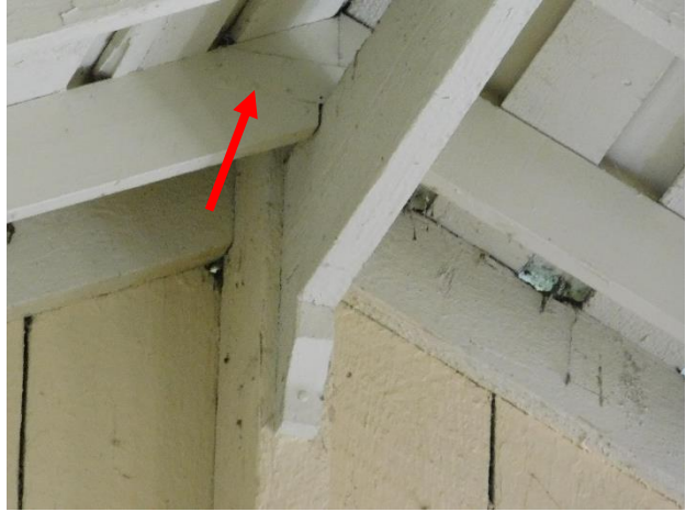
Figure 67. Corbel detail at ends of ridge beam. Also note the strapping at the ridge of the new additional rafters for the reconstructed belfry (arrow).
