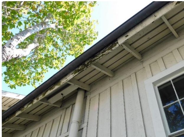
Figure 53. Example of loose and missing paint at roof framing.
