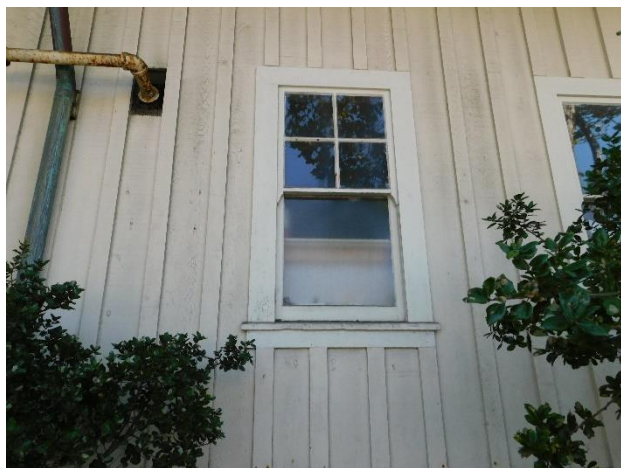
Figure 31. A 4/1 double-hung wood window at the men's bathroom.
