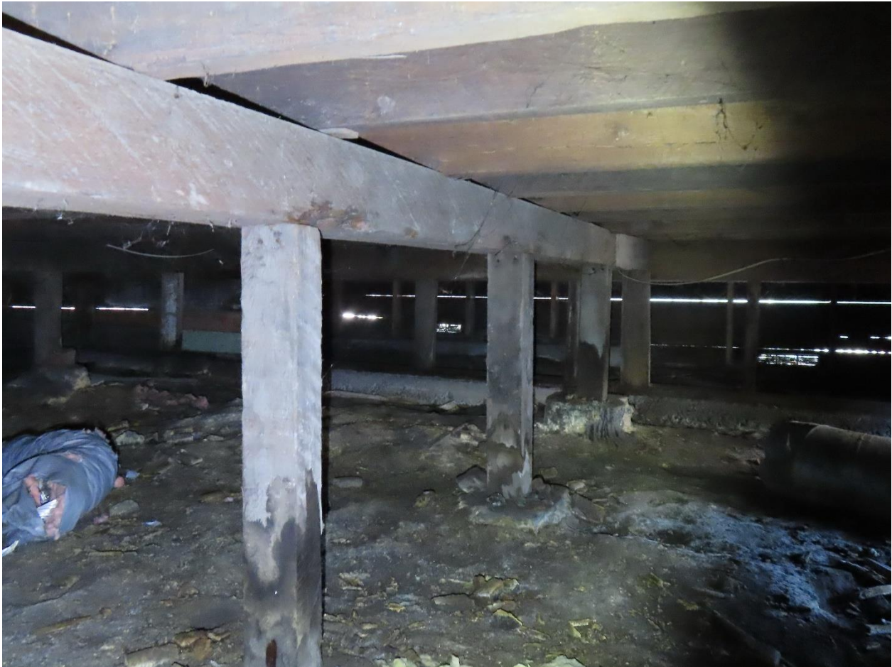
Figure 92. Water staining and damp soil in the crawl space of Chautauqua Hall.
