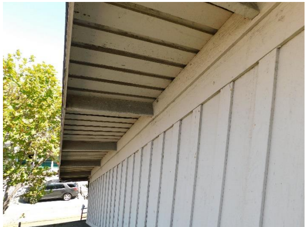
Figure 49. Exposed roof eaves, framing, and skip sheathing.
