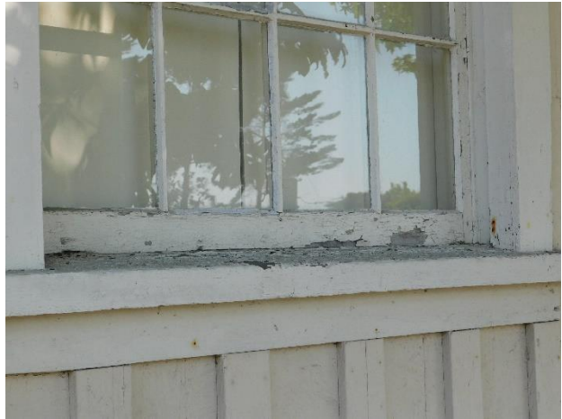
Figure 34. Deterioration and peeling paint at bottom rails of sashes and at window sills.
