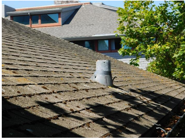
Figure 51. Biological growth seen at shaded areas of the roof and a missing cap over the large vent.
