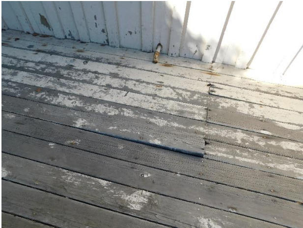
Figure 16. Loose deck board at the south deck.
