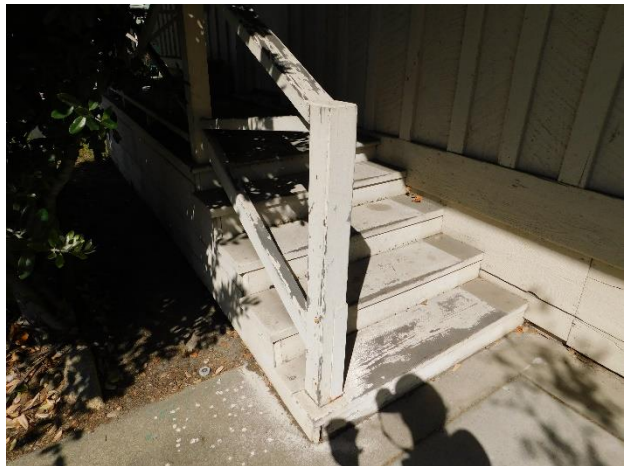
Figure 19. Example of loose, flaking, and missing paint at painted wood elements, including walking surfaces.
