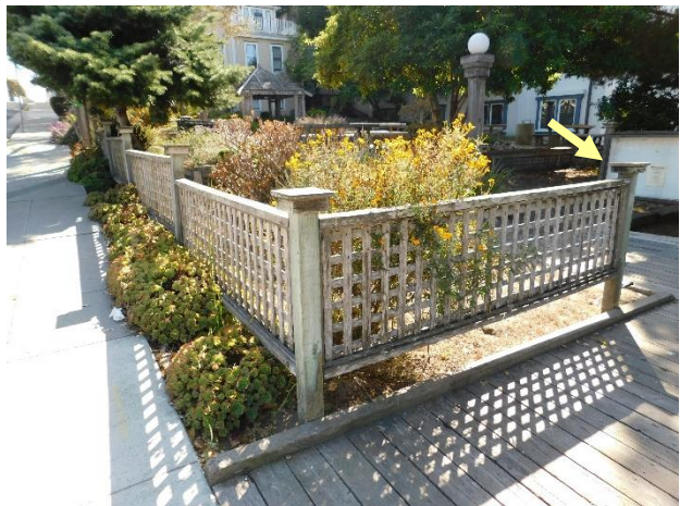
Figure 21. Loose garden wall post (arrow).
