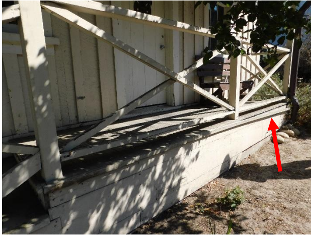
Figure 22. Loose skirting trim at a west porch (arrow).
