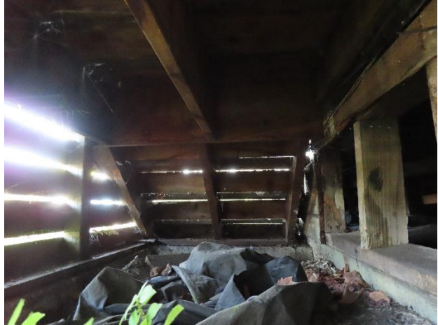
Figure 15. Framing and foundations beneath the north landing and stair.
