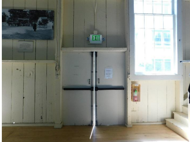
Figure 44. Daylight between a double-leaf door in the main hall.
