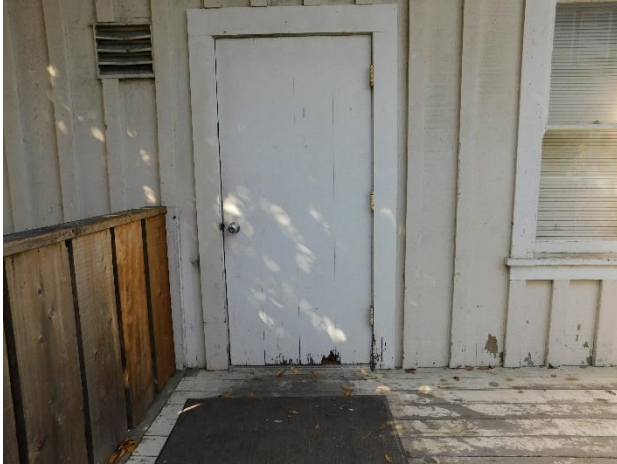
Figure 43. Deteriorated paint and wood boards at the bottom of an exterior wood door.
