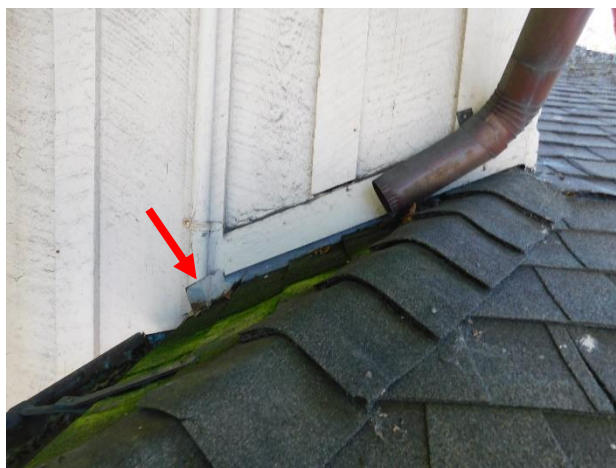
Figure 57. Sidewall flashing with kick-out (arrow) at north wall of main hall. Also note the exposed roofing nails at the hip shingles.
